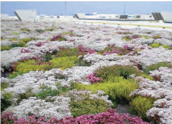
Green roofs reduce heat island effect, use rainwater and provide additional park space
