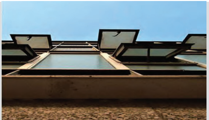
Increased ventilation will take advantage of winds coming off of the water for cooling during the hot Boston summer
